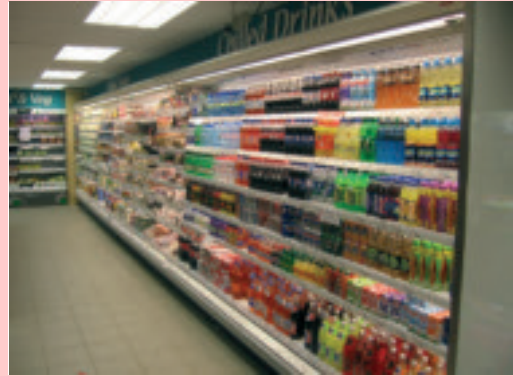
More refrigeration will boost sales of chilled products.
